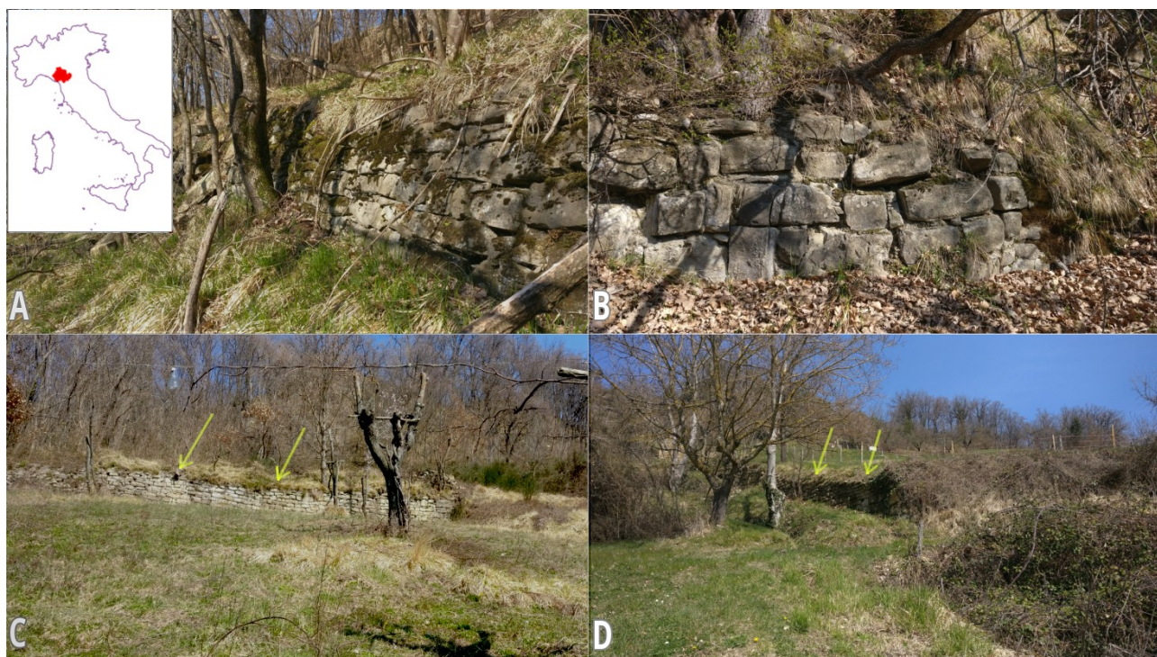
Figure 1. A and B: examples of abandoned historic agricultural terraces preserved beneath afforested canopy cover. C and D: examples of similar stone walls built between steeply sloping fields and along routes (yellow arrows).
