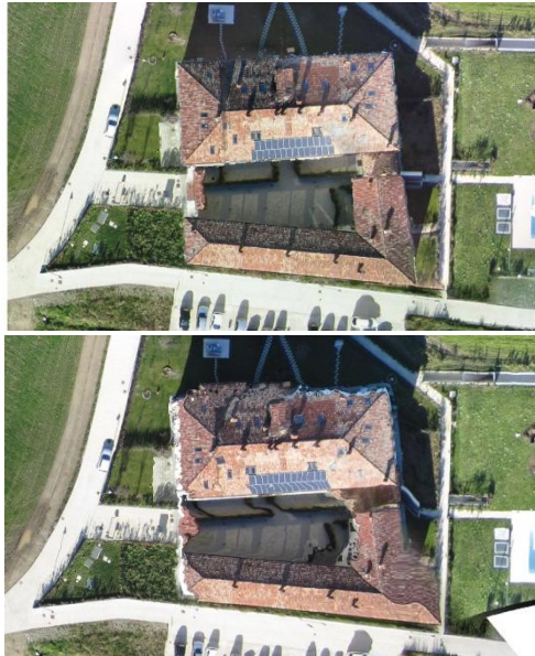
Figure 9 - Differences of orthophotos (AP up - P4 down): detail in the edges of some buildings
