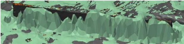
Figure 10. Retaining wall of the overflow area 3 of polder 2, UAS-DSM in green and TLS-DSM in gray (perspective view from the south)
