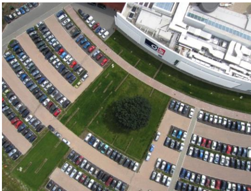
Figure 6: RPAS image of OS headquarter building.
