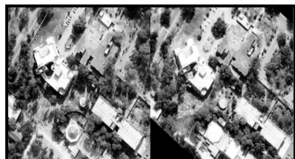
Figure 5. Aerial Image (left) and Google Earth Image (right) of Department Office Building in IIT Kanpur
