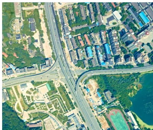
Figure 1. Overview of the Zhuodaoquan Viaduct
