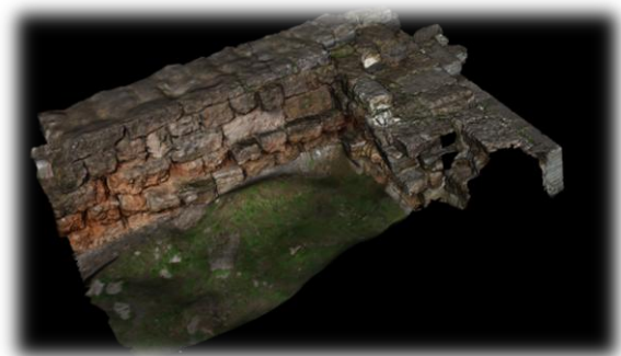
Figure 5: The 3D textured model of the foundations
