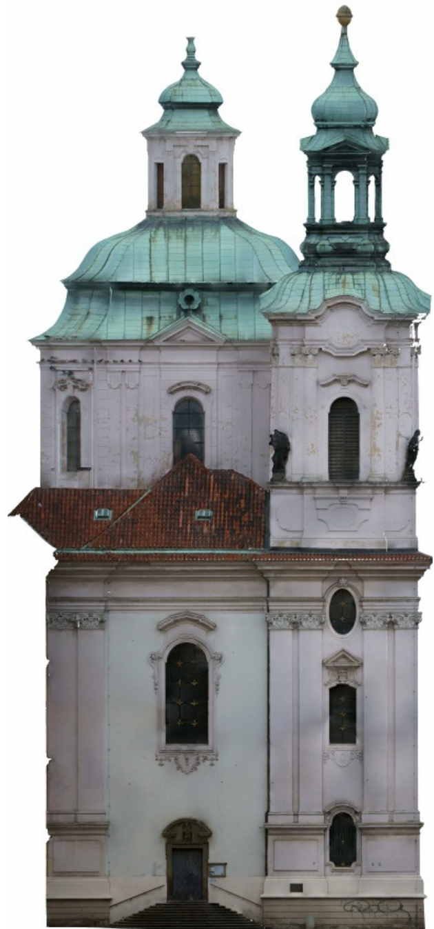
Figure 7. Orthophoto of west facade
