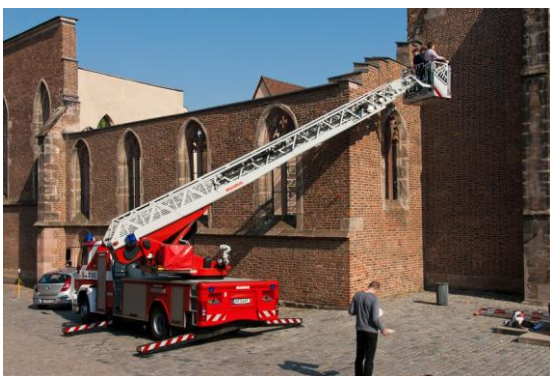
Fig. 3 Placement of photogrammetric survey markers around the building – supported by supported by the fire department of the city of Nuremberg
