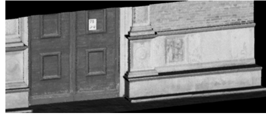
Figure 7. Laser scanner reading of the benches on the facade
