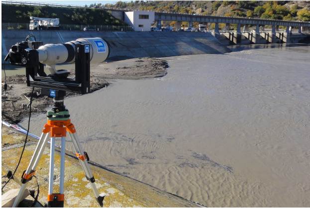
Figure 6. High resolution camera, 600 mm lens and panoramic head facing upstream wall of a dam
