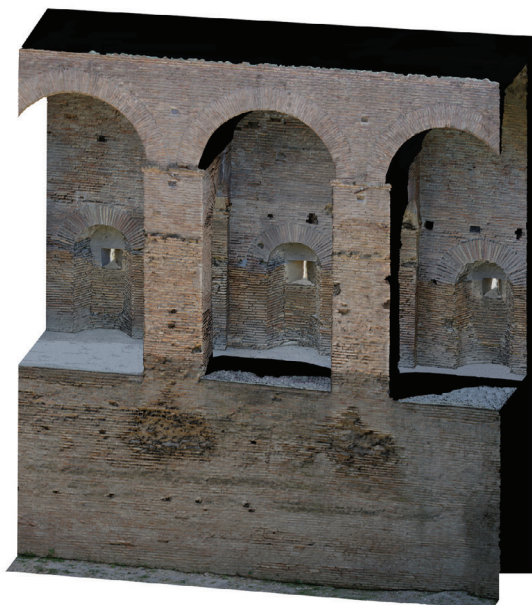
Figure 4. portion of 3D model: color projection on the triangulated surface.
