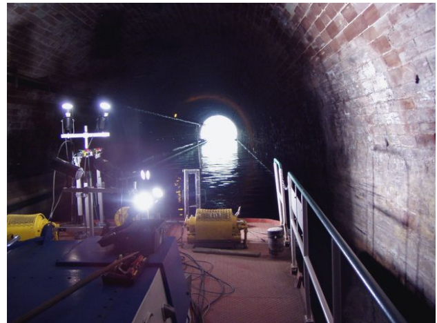
Figure 7: Modular imaging prototype onboard a barge in the experimental tunnel.
