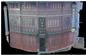
Figure 14. The color point cloud model of the building of Fulintang in Wenming Block
