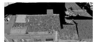
Figure 13. The three-dimensional (3D) point cloud of the roof
