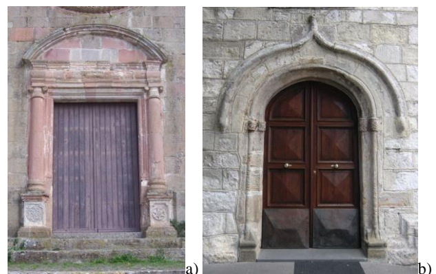
Figure 3. Example of portals: a) lintel (influenced by Italian Renaissance), San Mauro, Sorgono (Nu); b) arch with three centers and “flame arch”, San Vincenzo, Orroli (Ca).
