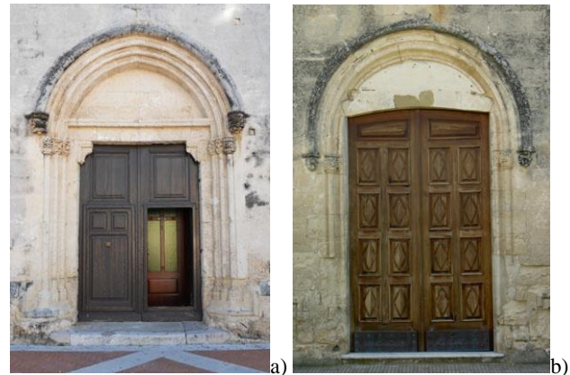
Figure 2. Example of portals: a) pointed arch, San Pietro Assemini, Ca; b) round arch, Beata Vergine Immacolata, Barumini (VS).
