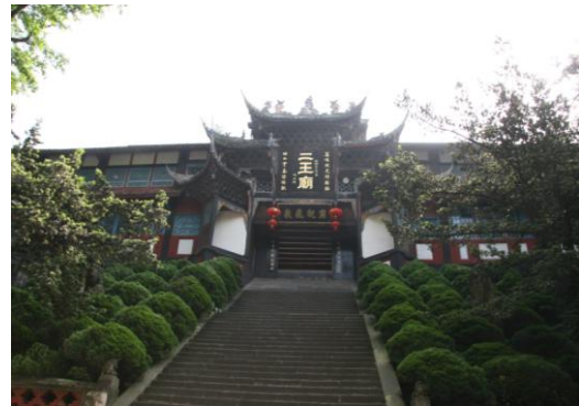
Photo 1. The picture of the stage before Wenchuan earthquake
