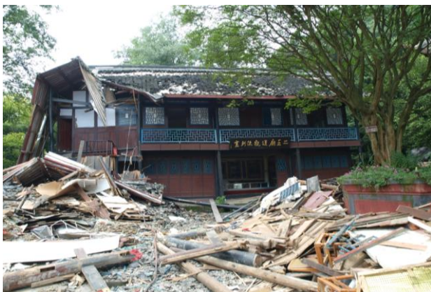
Photo 3. The picture of west guest room after the earthquake
