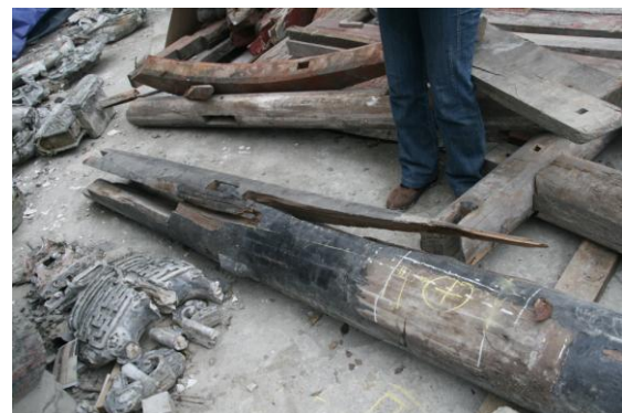
Photo 5. The component which may continue to be used by strengthening and maintenance
