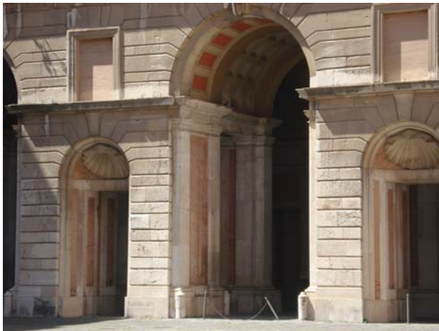
Figure 7 . Courtyard of Royal Palace in Caserta
