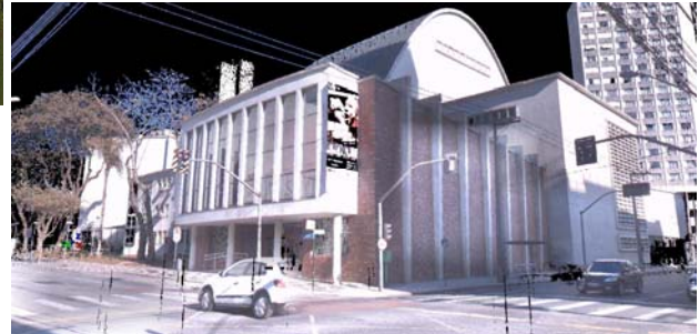
Figure 11. Image Texture Map on Point Clouds: structural faults and tiny cracks on walls were not visible
