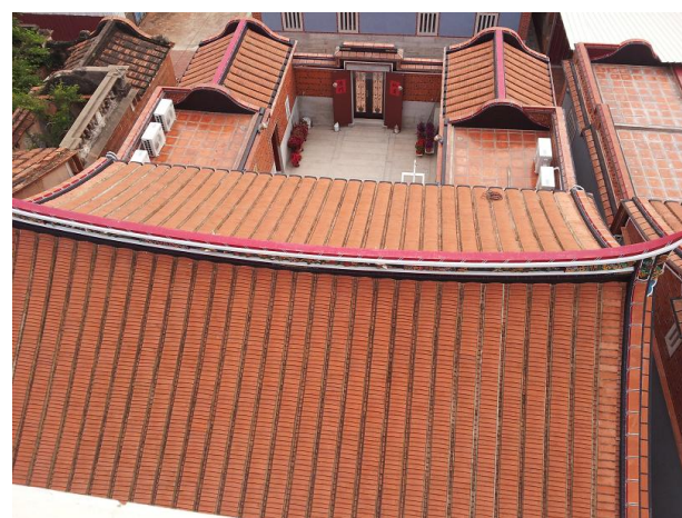
Figure 2. Residential house in Jinning Town, Kinmen County
