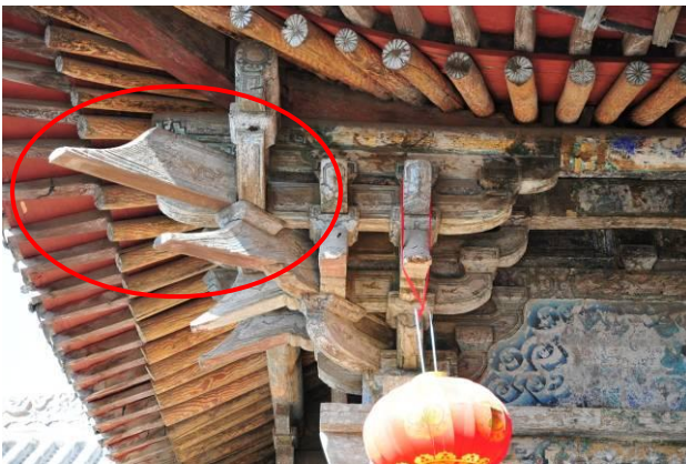
Figure 9 “qin mian ang” with a gently curved arc
