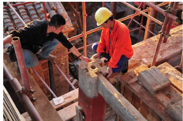
Figure 12 beam not really comes out at the corner
