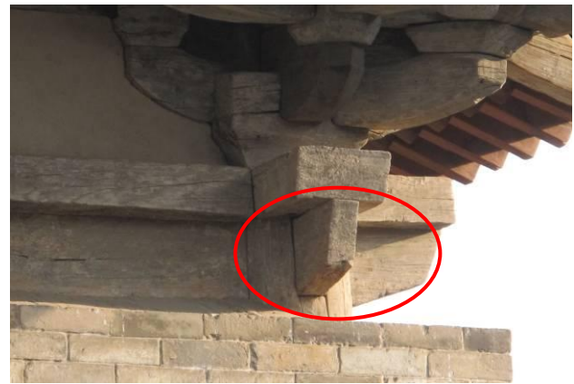
Figure 11 beam head comes out at the corner
