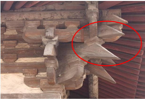
Figure 8 “pi zhu ang” with a straight slope
