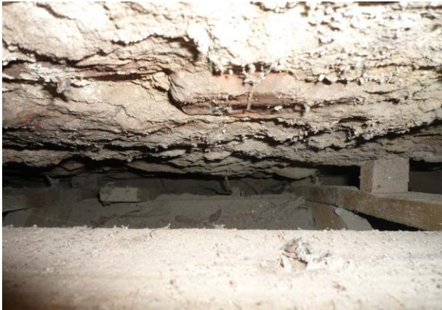
Figure 3. View inside the cavity wall before insulation
