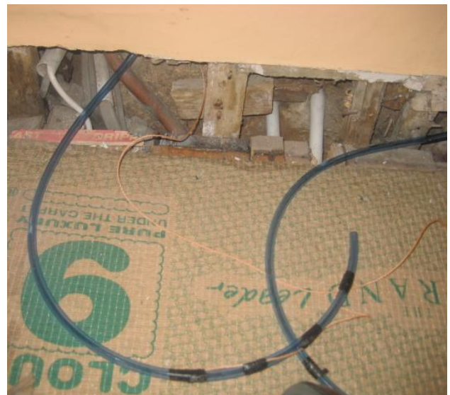
Figure 9. Pipes attached to cords
