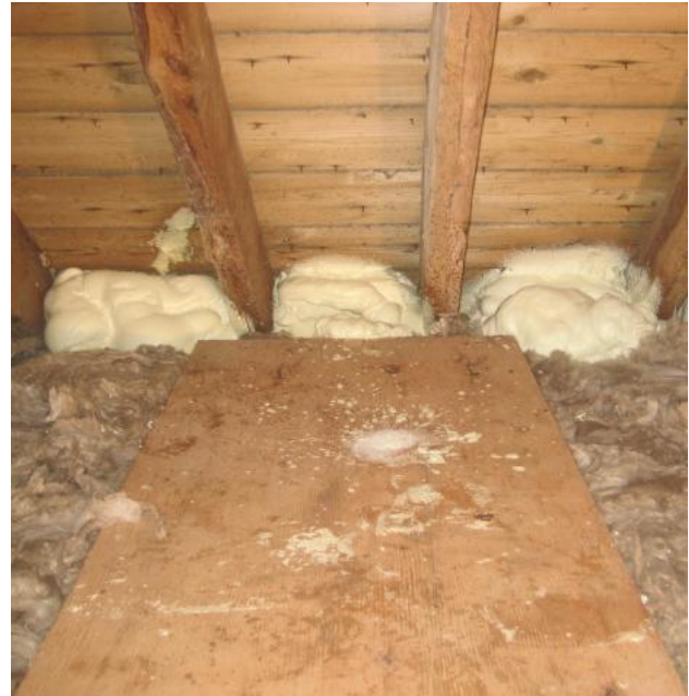
Figure 18. Foam seen at the eave level
