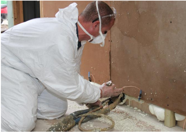
Figure 6. Injection of the foam
