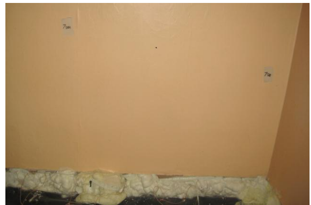
Figure 14. Leak of the foam at the bottom pat of the wall
