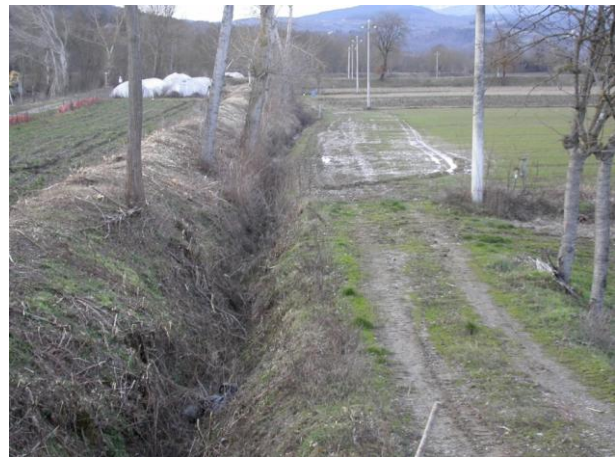
Figure 14. Example of drainage ditch
