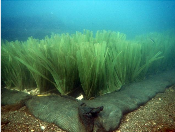
Figure 6. An artificial seagrass mat on the seabed. The plastic fronds work in two ways; catch sediment suspended in the water column and create a burial mound or if there is no sediment transport they can slow down water currents.
