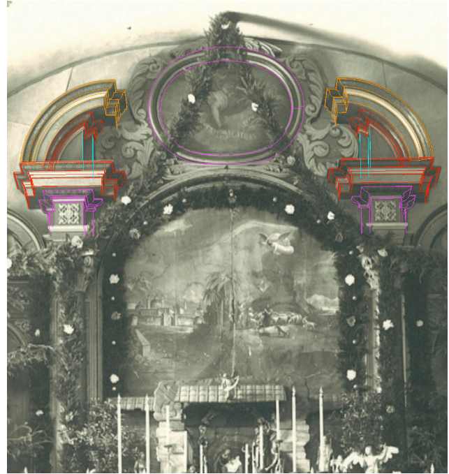
Figure 8: Rigorous audit by back projection of the reconstructed outlines into historical photo 2
