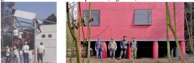
Figure 9. Left: the assembly of this lightweight building system in Xiasi project.
