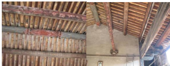
Figure 11. Central Beams and Lamp Beams
