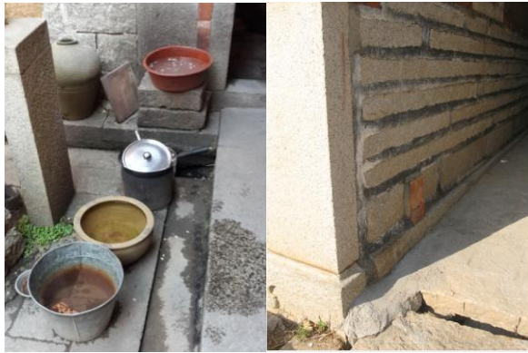
Figure 9. Drainage outlet of patio and cat alley
