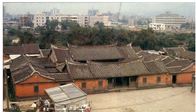
Figure 2: The Lin-An-Tai historic building in 1977 (Gan-Lang Li, 1977).
