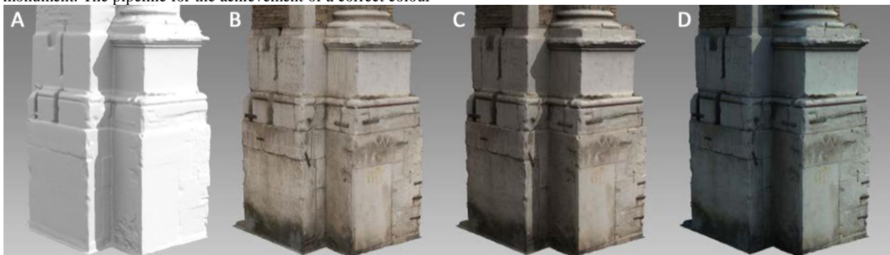
Figure 8. Detail of Porta Sisi: A) mesh shading (direct and indirect illumination); B) apparent colour used as luminous texture; C) and D) “double shadowed” model rendered under different lighting conditions.
