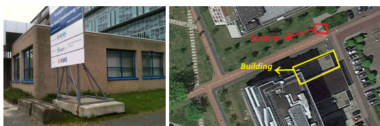
Figure 1: Left; the building chosen for our first showcase. Right; Google earth view indicating the location of the building of interest and the TLS scanner position.
