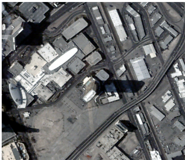
Figure 4. HRC Image of the Trump Tower in Las Vegas, Nevada
