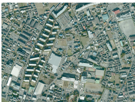
Figure 2. Aerial images in Saitama District year 2012
