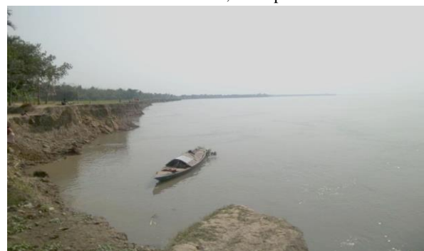
Figure 10. Bank erosion 6 km south from Bahadurabad.
