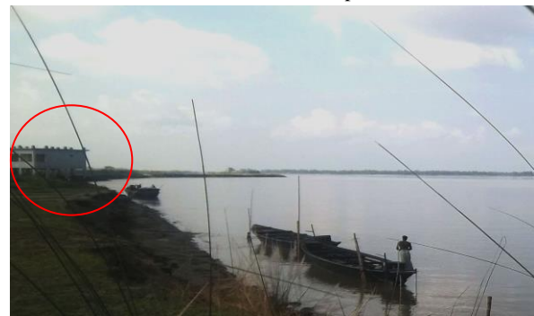
Figure 8. Govt. Primary School at Belgacha facing serious threat of bank erosion .
