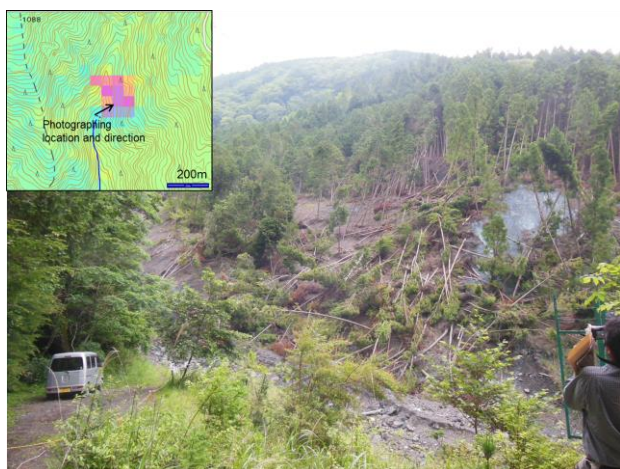
Figure 3. Field photo of landslide collapse in Shizuoka site (June 25, 2013).
