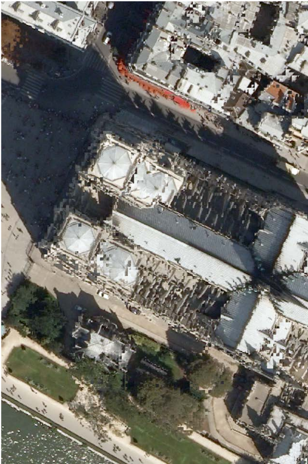
Fig. 12: True orthophoto on an irregular surface (gothic church roof with duplications etc.)
