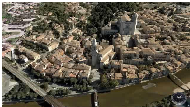
Figure 8: Photo-realistic 3D city model produced with oblique imagery with possible semantics and webGIS exploitations.
