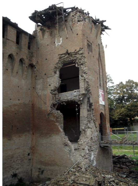
Figure 2. Seismic damages to the North Tower of the San Felice sul Panaro Fortress
