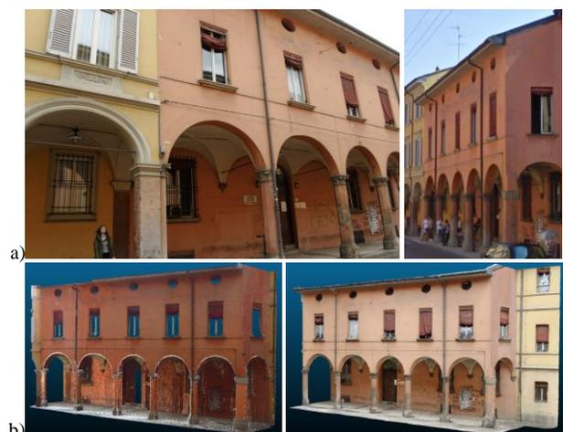
Figure 4: The building with porticoes used for the reported assessment (a). Result of the range-based (b-left) and image (b-right) 3D surveying.
