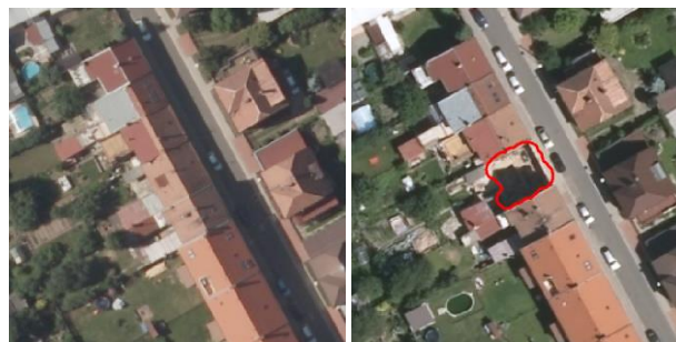
Figure 6. True indication of a demolished building
