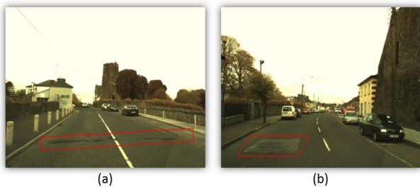
Figure 4: Digital image of (a) first and (b) second section of urban road with roughness regions indicated in red boxes.
