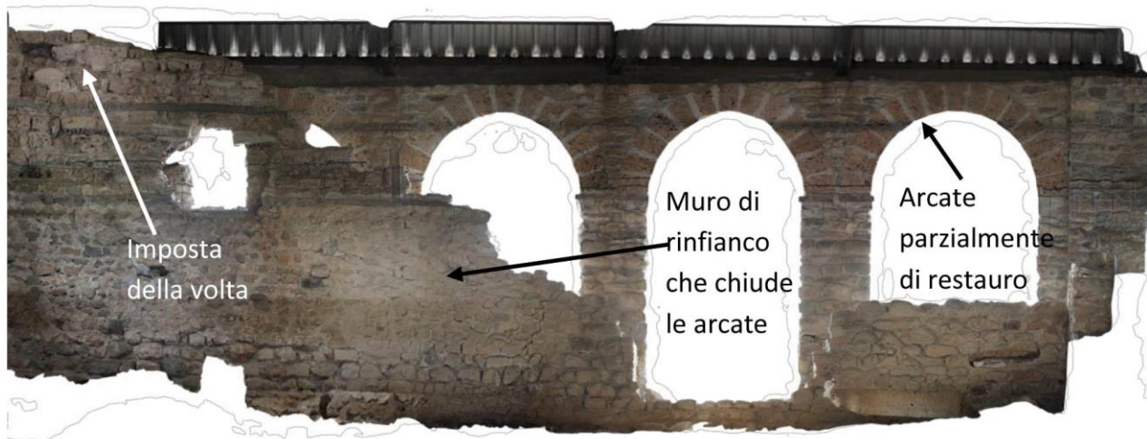
Figure 2. Laser-scanner survey of the late ancient arches (Politecnico di Milano).
