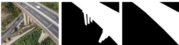
Figure 9. Annunziata Viaduct from UAV Photo (a), and 2d masks of the bridge (b) and deck (c)
