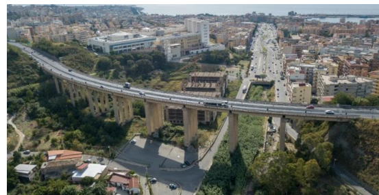
Figure 6. Annunziata Viaduct in A2 highway
