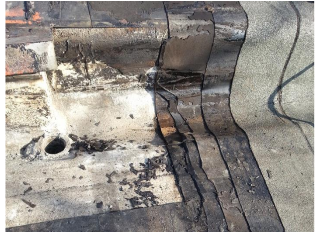
Figure 4. Non-accessible roof (Ambrosini's photo, 2016)
