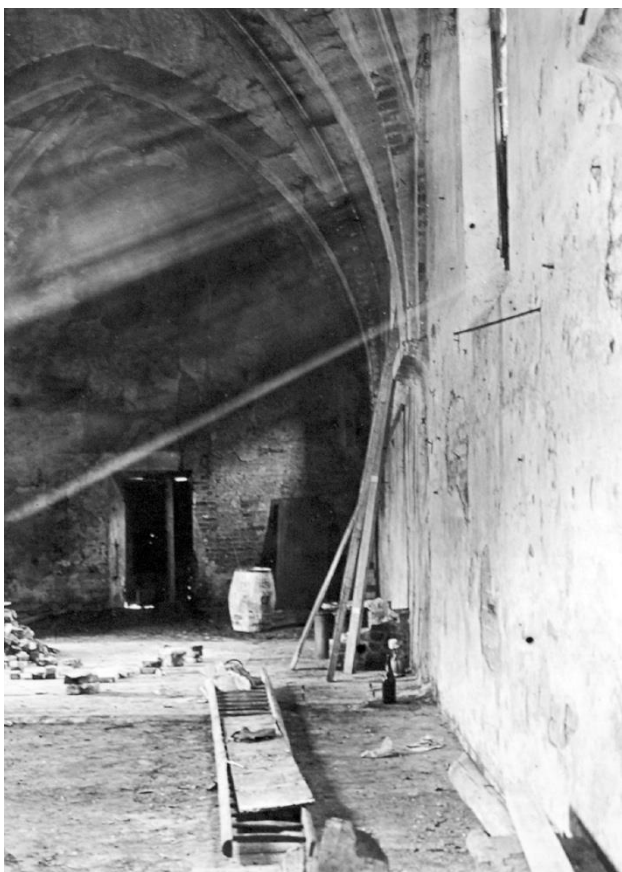
Figure 11. The interior of the Refectory in a picture that documents the state of consistency before the restoration of Ferdinando Reggiori. On the back wall there is still the door then closed and the walls are plastered. Therefore, the photo dates back to the beginning of the works carried out by Reggiori (fig. 12) (AACMi)
