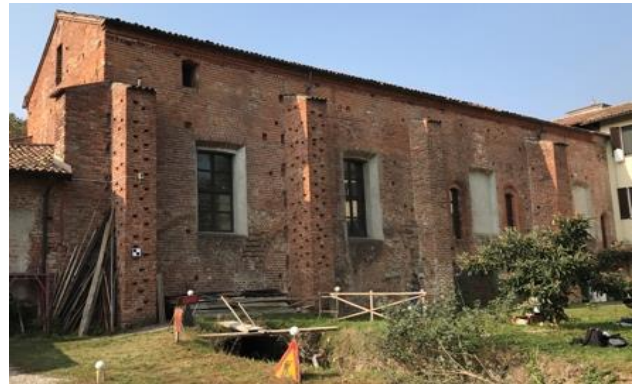
Figure 22. Photo of the eastern front of the Refectory with the canal in the foreground (photo October 2017)
