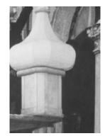
Figure 3. Basic model for a 3D shape reconstruction of a cupola on lantern. Scale 1:5, placed on scaffolding at a relative height © Boris Lobovikov archive
