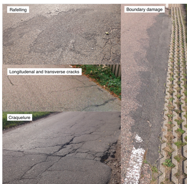
Figure 1. Examples of road surface damage.
