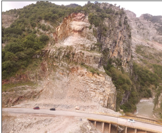
Figure 3. Panoramic view of the landslide case site in Proussos area, Greece
