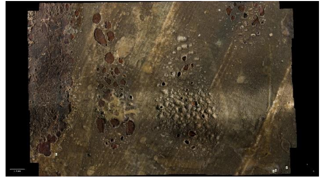
Figure 8. St. Constantine and Helen: area characterized by blisters and flaking. Orthomosaic
