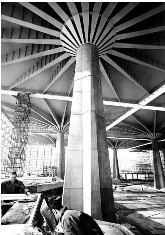
section at the top. In order to be able to model the pillar, it was
