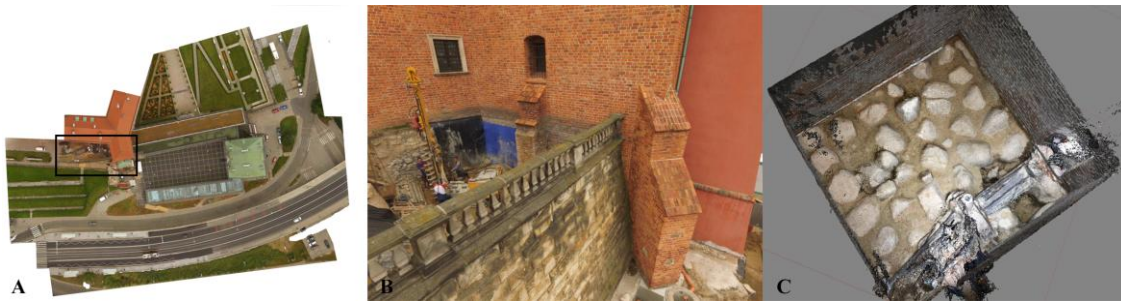
Figure 2. A) A section of a true-orthophotomap with the excavation area marked; B) example of the exterior excavation; C) the analysed interior
