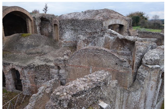
Figure 2. Picture showing the complex shape of Small Baths' roofing made of intersecting volumes.
